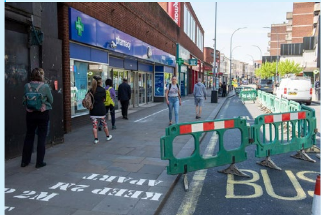
Figure 1: Footway widening scheme in Hammersmith and Fulham, London
